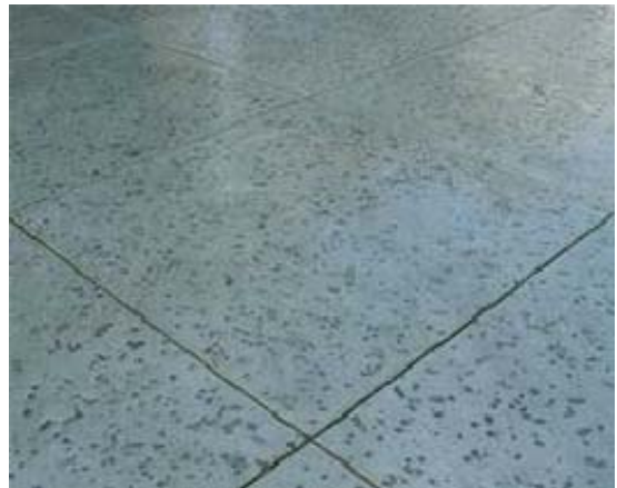
Concrete Deck Blue-Gray, rock salt finish
