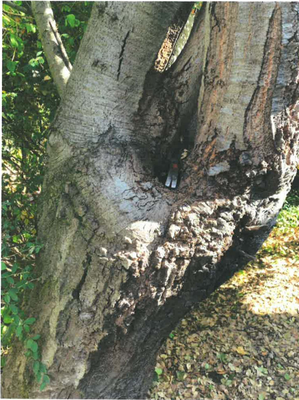
Figure 2. Decay cavity in the common attachment of the codominant spars. Framing hammer inserted in the cavity visible in the center of the image.
